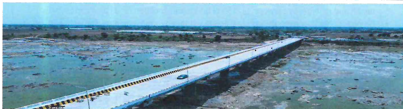
Aerial view of Barana-Jalwara-Nahargarh bridge
