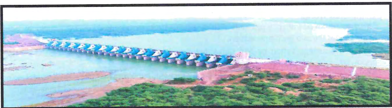
Navnera Barrage Project, Kota
